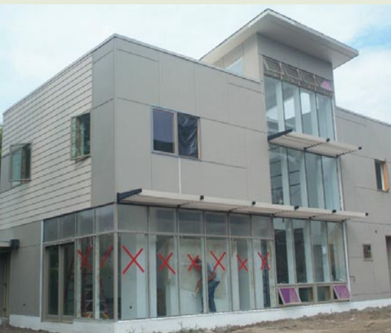
[Above left] Eva Kultermann, College of Architecture faculty member, puts some finishing touches on a window inside the green home.
